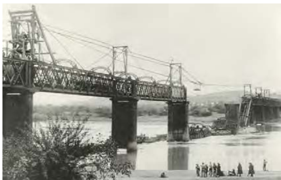
Among projects on which Lieutenant-Colonel Parrott worked during the Anglo-Boer War was the repair of the Norval's Pont Railway Bridge across the Orange River, which retreating Boer troops had dynamited in March 1900. A temporary pontoon bridge was put in place by the Pontoon Troop of the 47th Company of the Royal Engineers, enabling foot soldiers to cross the river.
