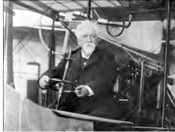
Hiram Maxim at the controls of a famous but impractical invention—his steam-powered, rail-mounted biplane made of tubular steel and canvas biplane in 1894. It 'flew' for about 200 metres during a trial in 1895 but then broke an axle and was so seriously damaged that Maxim abandoned the project.
