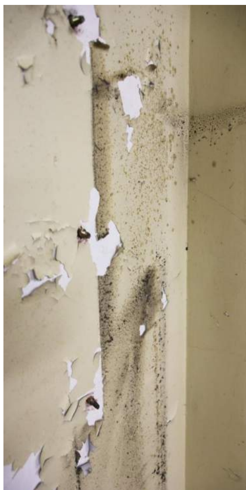
This corner harboured a dead air pocket and trapped moisture, causing black mould to form and the paint to peel.
