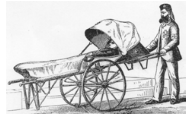
The St John Ambulance Litter about 1874. It was modelled on the ‘Neuss’. Who designed it is uncertain, but possibly it was the litter for which Surgeon-Major William GN Manley, VC received ‘Letters Patent’ in 1875.
